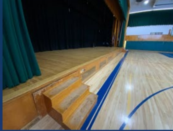
Auditorium Stage Refinishing / ADA Access
