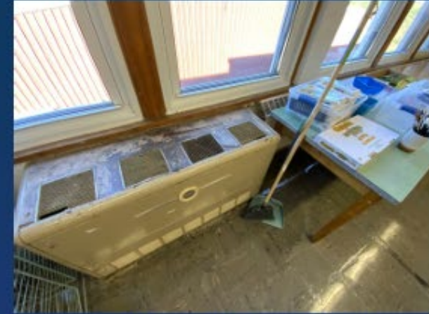
Unit Ventilator Replacement
