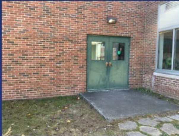
Door Replacement / HW Upgrades
