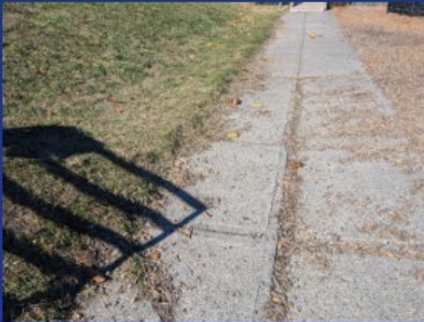
Reconstruct Asphalt and Concrete
