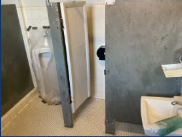
Plumbing fixture / Facility Upgrades
