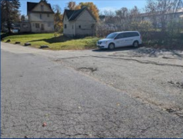
Reconstruct Asphalt and Concrete
