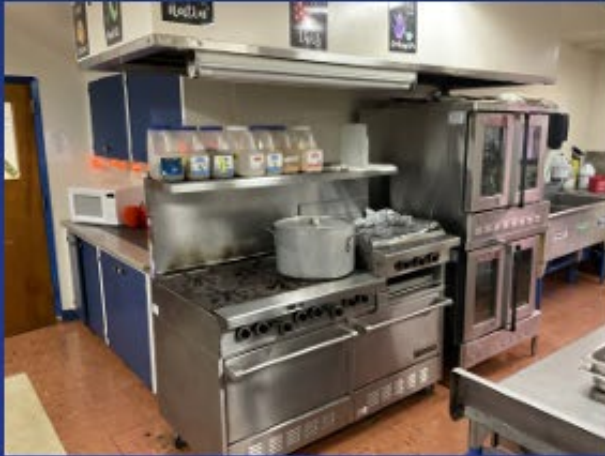
Kitchen Hood Replacement
