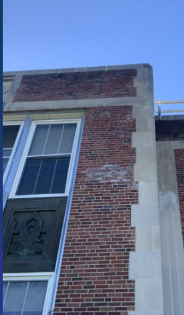
Repointing, Masonry Cleaning
