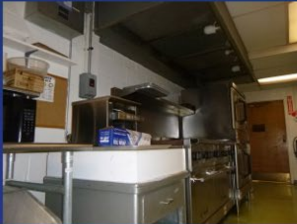
Kitchen Hood Replacement
