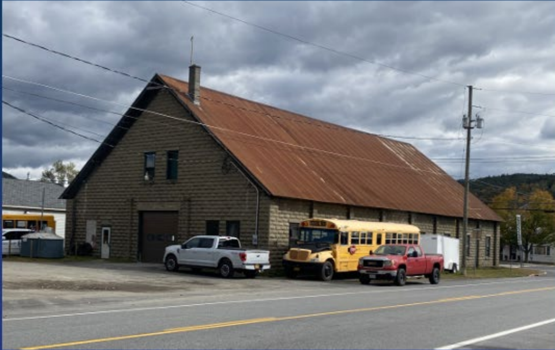
Metal Roof Replacement / Exterior Masonry Renovations
