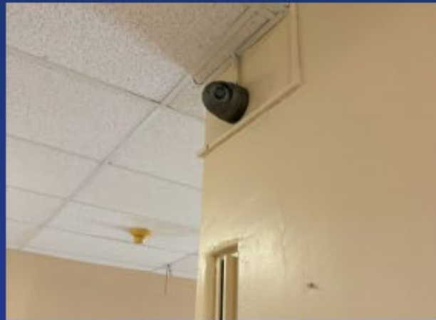
Fire Alarm / CCTV Upgrades
