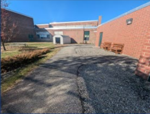
Reconstruct Asphalt and Concrete Sidewalks
