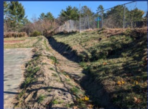
Stabilize Drainage Swale
