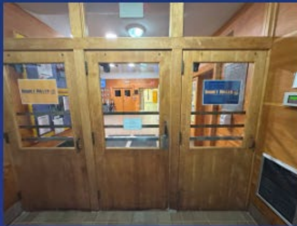
Secure Vestibule Upgrades
