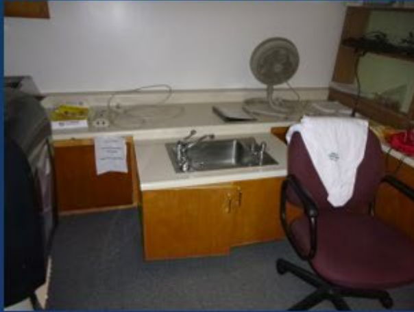
Plumbing fixture / Piping Upgrades
