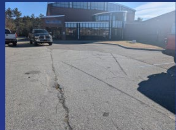
Parking Lot Reconstruction
