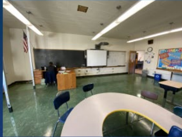
Hazardous Material Present Throughout (Floors, Ceilings, Chalkboards)
