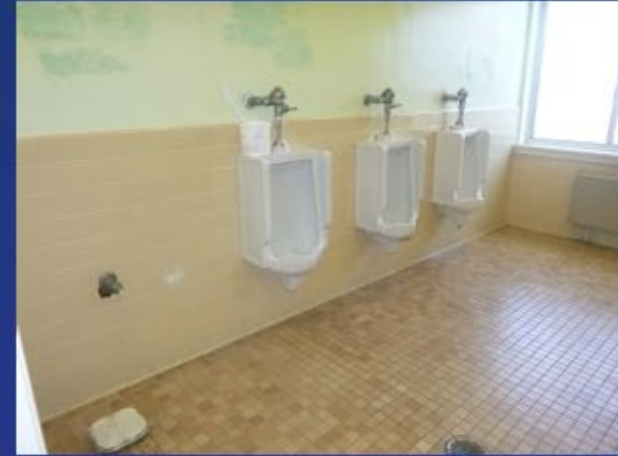
Gang Bathroom Upgrades Fixtures / ADA Accessibility
