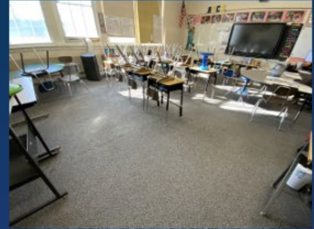
Carpet Replacement (assumed over VAT)
