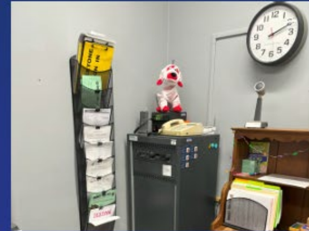
PA / Clock System Upgrades
